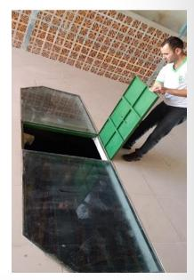
Rainwater capture system with capacity to store 100 thousand liters of water installed at Rectory. Use of water in toilets and irrigation of gardens.
